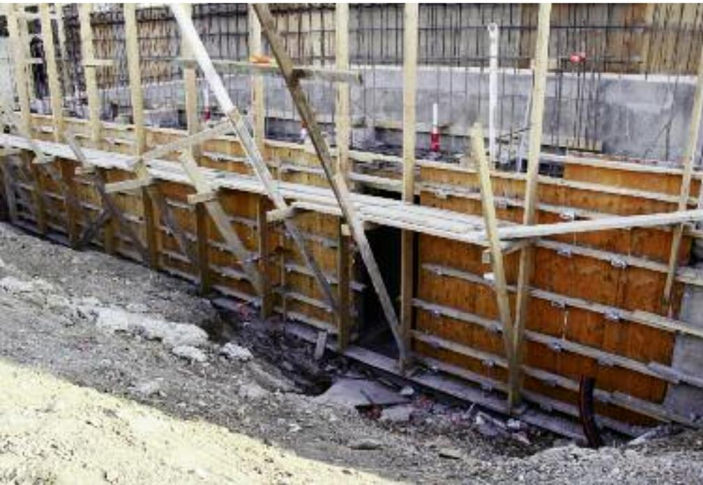
The construction processes followed with poured-in-place concrete allow a measure of precision that is much harder to come by when using pneumatically applied material – a wonderful advantage when it comes to executing rectilinear designs and all-tile finishes because the walls are so amazingly clean when the forms are pulled.
